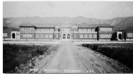
Burbank High School Paving Project Before
